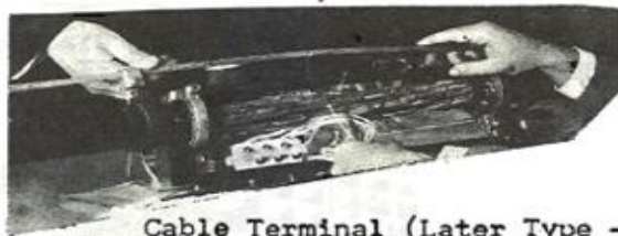
Cable Terminal (Later Type - Mounted on Cable instead of Pole.)
